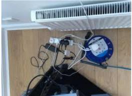
• Proprietary purpose designed, and manufactured desks leads can be used to comply with the current BS 6396 (**See picture below**)
